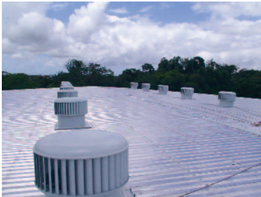
FIGURE 6.5 Installation of Hurricane H900HI Ventilators
